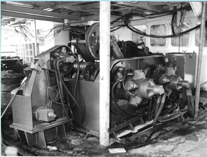
The impressive hydraulic pipework of the new traction winch.
